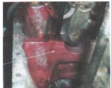
Fig 3 After wiping off most of the dye and applying the developer, the crack is clearly visible as a red line
